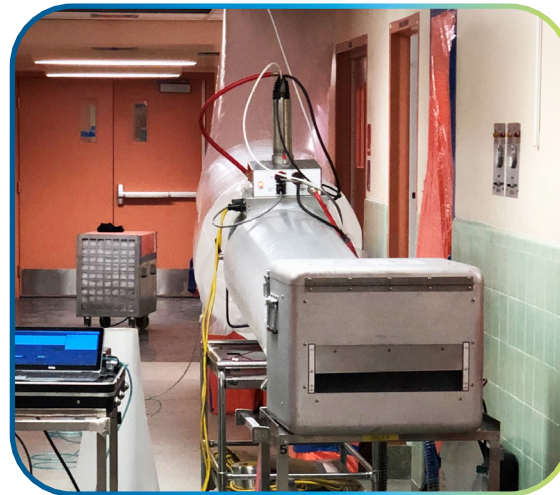
Aeroseal Equipment Sealing Ductwork
