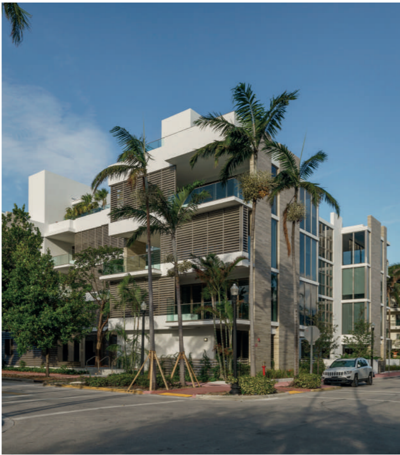
Louver House, Miami, USA
