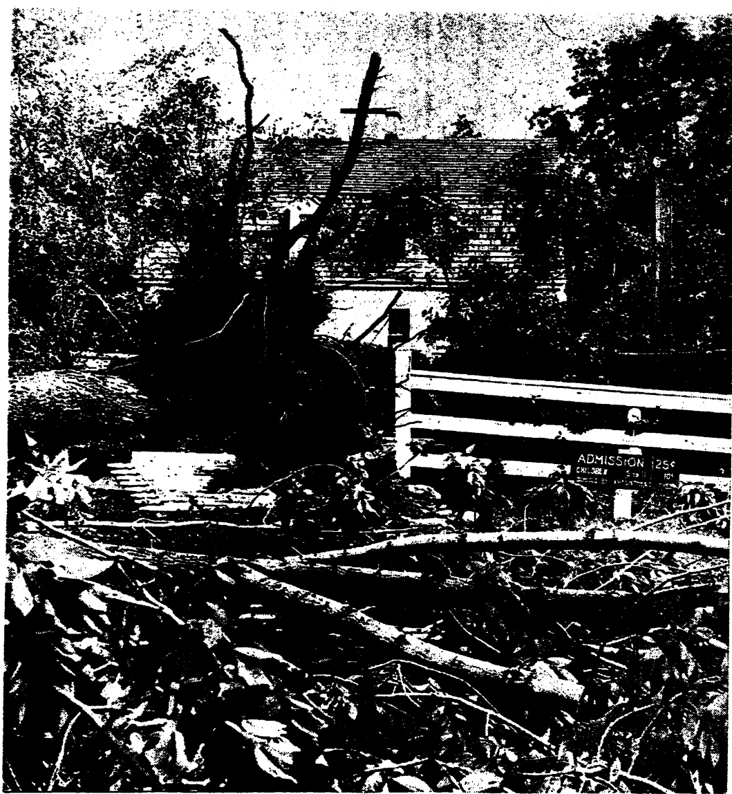
FERRY HOUSE SAFE AMID STORM-RIPPED TREES: Some two dozen trees clustering about historic McKonkey's Ferry House (above) in Washington Crossing State Park were blown down in the tornado yesterday afternoon.
