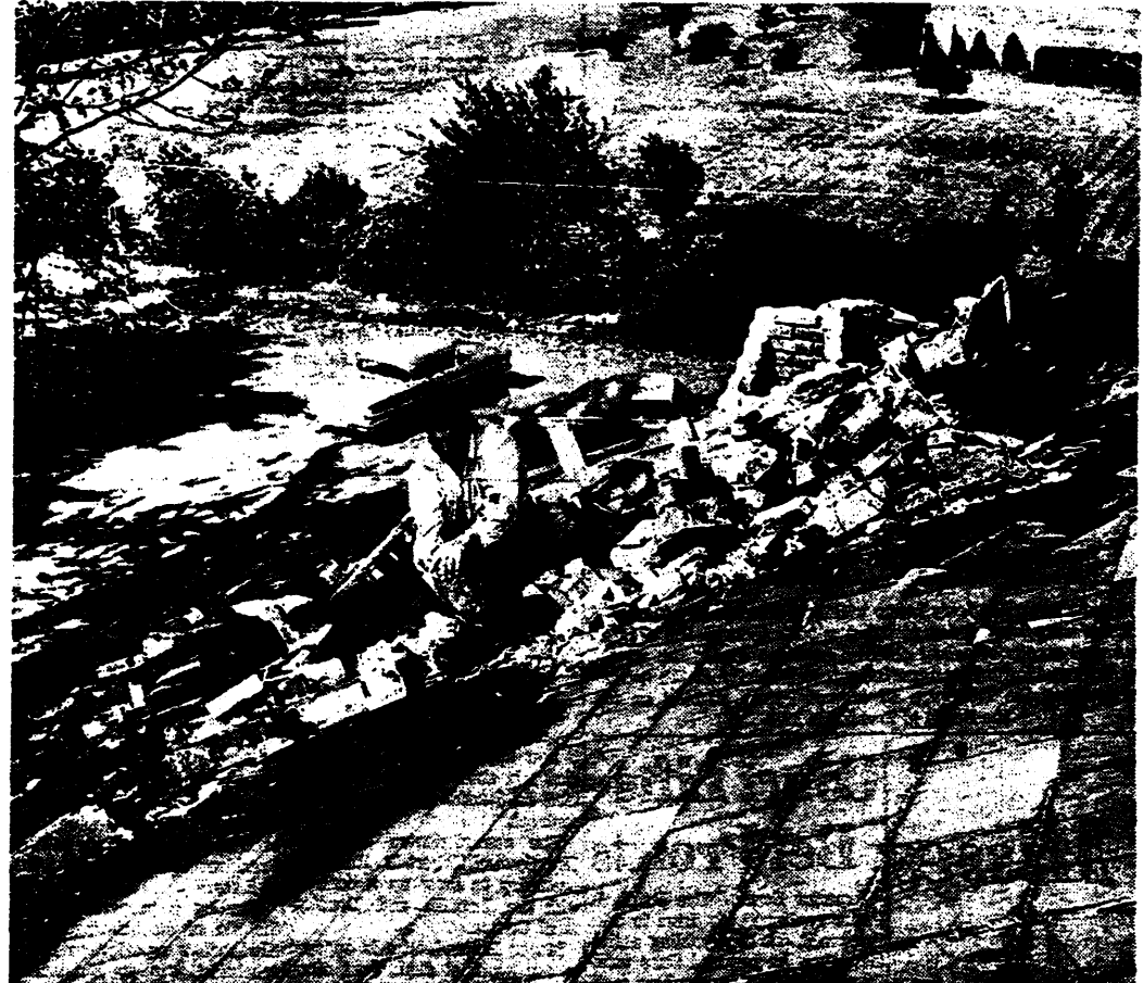
A huge tree, blown over by the wind, smashed chimney through the roof of the Chapin School on Princeton Pike. The school was severely damaged by the storm.
