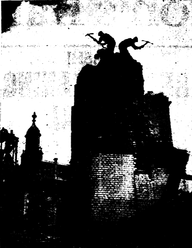
LONDON, July 7.—These two men are knocking down, almost from under their feet, the shattered structure of a blitzed building in Fetter Lane. Theirs is the most dangerous part of demolition work after raids.
